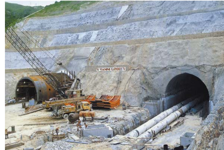
Junk Bay Tunnel
