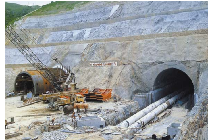
Junk Bay Tunnel
