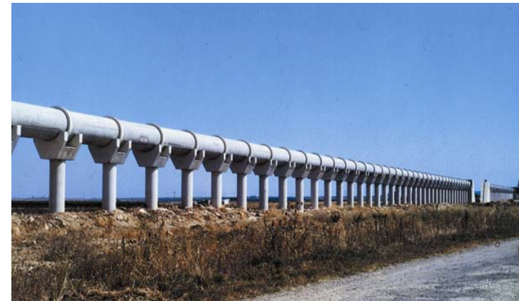
Pertusillo water infrastructure
